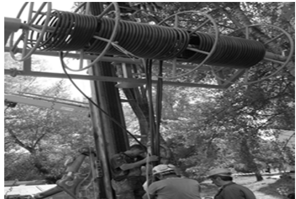
Fig.8. Inserting the HDPE tubes in the perforations
