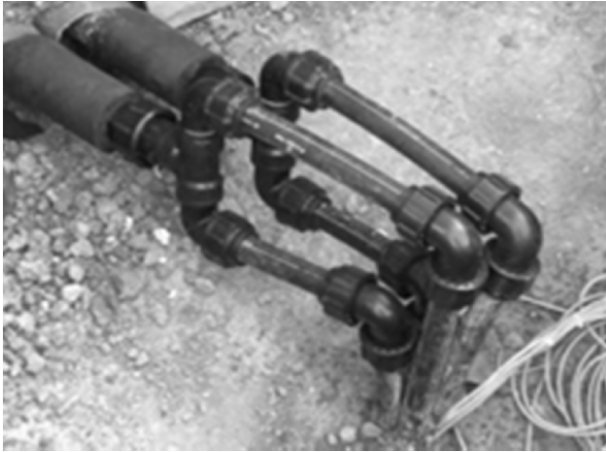
Fig.9. Upper part of the double U-tube borehole
