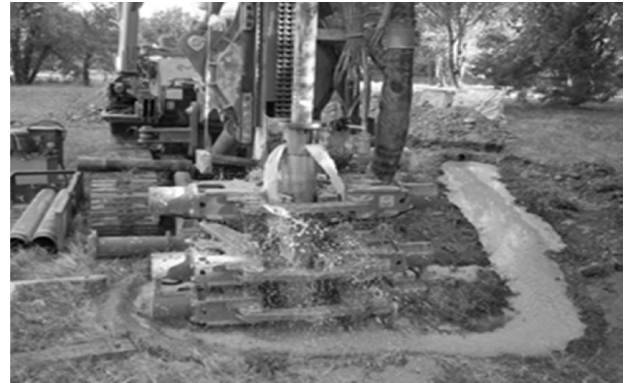
Fig.7. Drilling of boreholes with MDT Mc 200 B
